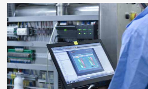
Equipment Assembly and Debugging
